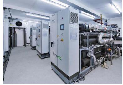
heat buffer storage connected with the heat pump evaporators. Because of the closed waste water circulating loop no special measures to avoid corrosion are necessary.
