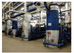
In parallel, other alternatives for the heating were assessed like a central gas fired boiler, combined heat power or geothermal heat pump. Qualitative and quantitative assessments (cost, required existing installation upgrade, future site growth...) defined that the best alternative solution for this project was the heat pump. So a correct analysis and understanding of the real need for the installation allow installing the right answer to the real Nestle needs.
